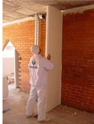
Figure 1. Operator disposing a plaster panel
